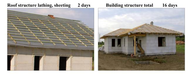
In ideal circumstances the building structure of a house with a floor space of  $100-120 \text{ m}^2$  is finished within 16 days. During the on-site assembly the engineering works can be commenced, so this technology reduces the time necessary for the construction works of the building.
